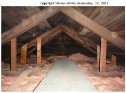
Recommendation if insulating at the ceiling: If the ceiling is not vaulted, all existing batt insulation should be removed. Then the overall insulation level in the attic should be 11+ inches of blown cellulose or fiberglass, which would result in a R-38+ to the ceiling plane. To do this in your attic, a couple things would need to be done.
