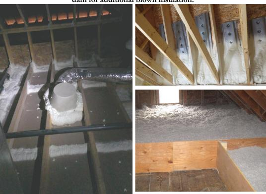
Recommendation if vaulting ceilings and insulating at the roof deck: There was discussion of vaulting all the ceilings where possible. In this case, it is recommended to use ccSPF against the roof deck to the full depth of the rafter and then cover with drywall to provide a fire rated assembly.
