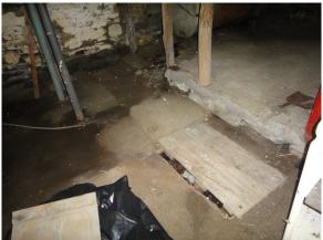
There is likely no below grade exterior water barrier on the foundation, so insulating the interior side of the foundation could result in water being trapped in the foundation assembly and deteriorating the integrity of the structure over time due to freeze-thaw. Exterior insulation options would require excavation around the foundation, which is limited on the front and left side of the home due to the porch and driveway.
